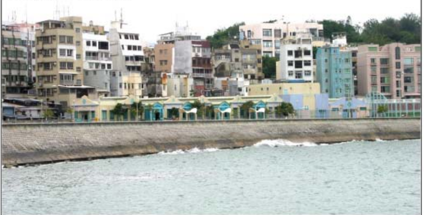
現狀 EXISTING CONDITION
